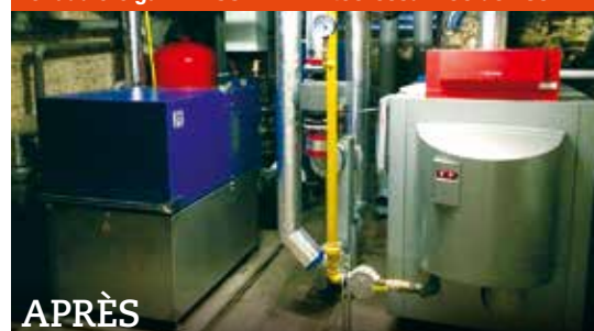
Chaudière gaz VISSMANN Vitocrossal 200 de 285 kW
